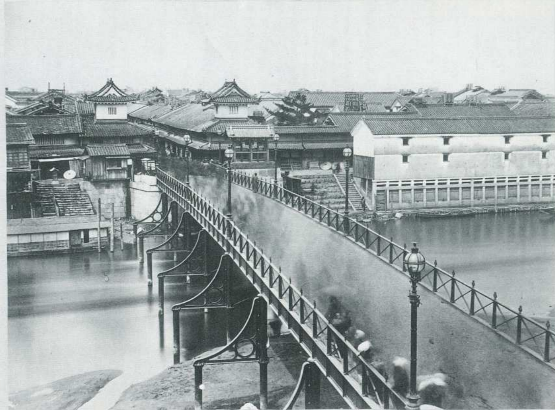
Osaka, Iron Bridge (Tetsuhashi).
